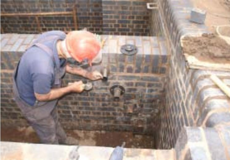
graduation of the base flow entering the canal to pass into Darnford Brook as demanded by the Environment Agency. Attention now turns to adding a blue brick facing to the concrete block towpath wall.
