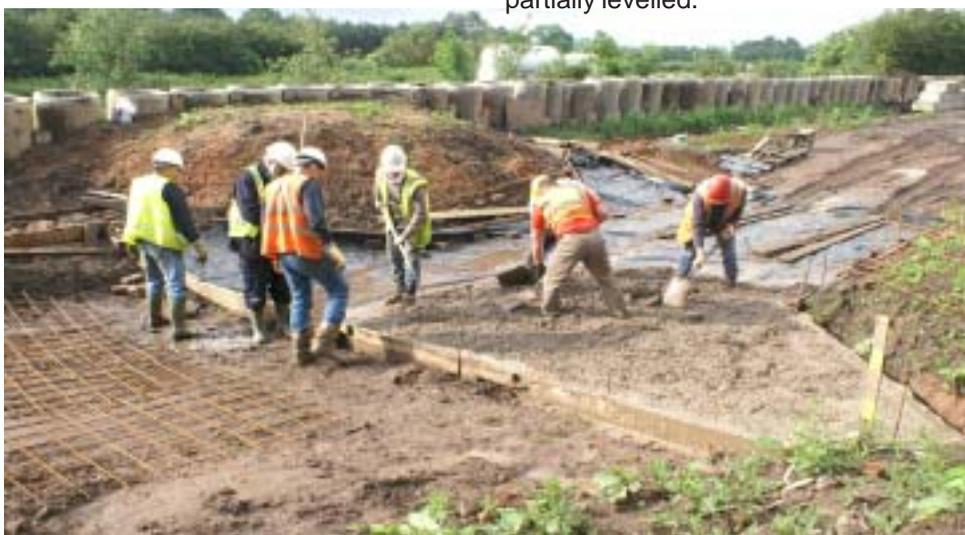
*Professional help laying the substantial concrete base to form the narrows*
