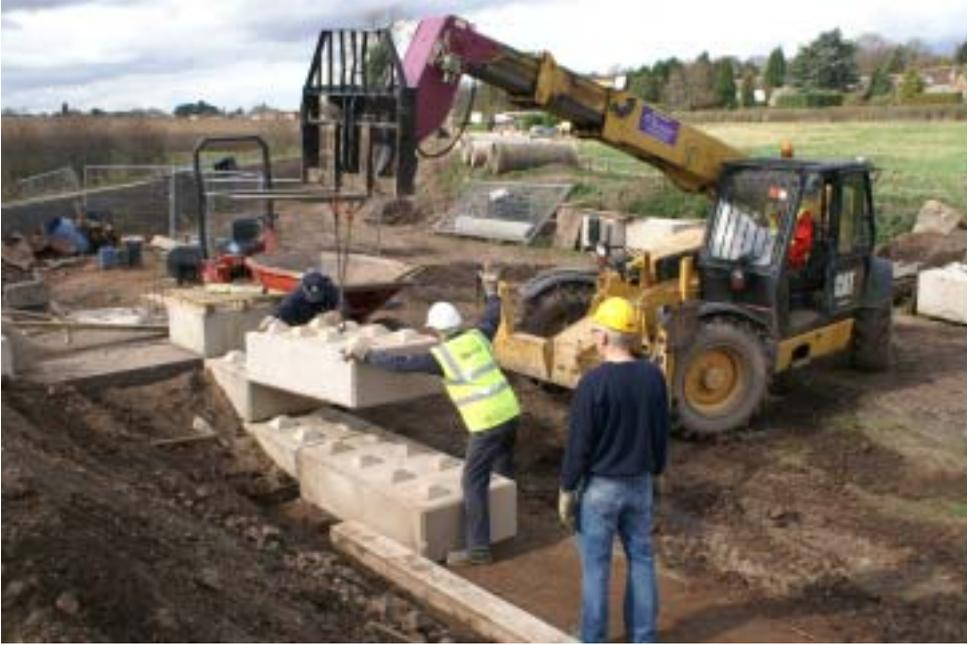
*Novel construction techniques used to build the new towpath wall in Pound 27, 17-Mar-12.*
