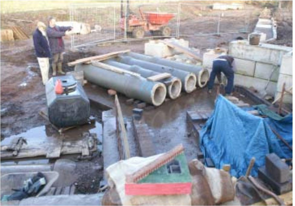
*Pipes laid in the new towpath will connect with the weir outlet, Jan-12*
