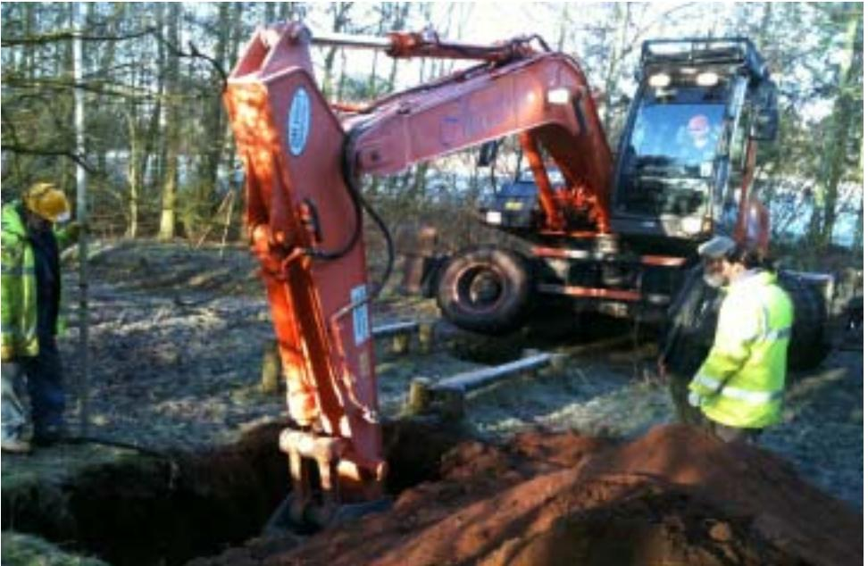
*One of the four trial holes dug in Darnford Park to test ground conditions*
