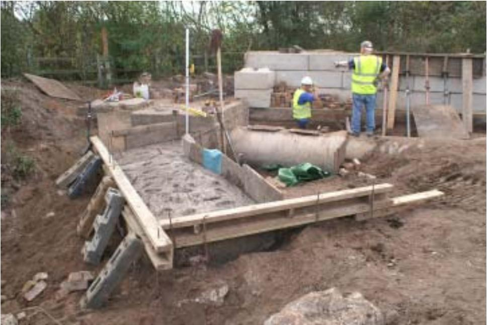
*Walls around the 'big pipe' at A38 corner will carry a weir to control the later outfall to the Darnford Brook, 2-Oct-11.*
