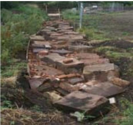
Further along Pound 27, foundations for the towpath wall are being extended along the section running in parallel with the A38. This needs to be particularly robust so a massive stone bed will carry the concrete base and upper wall structure.
