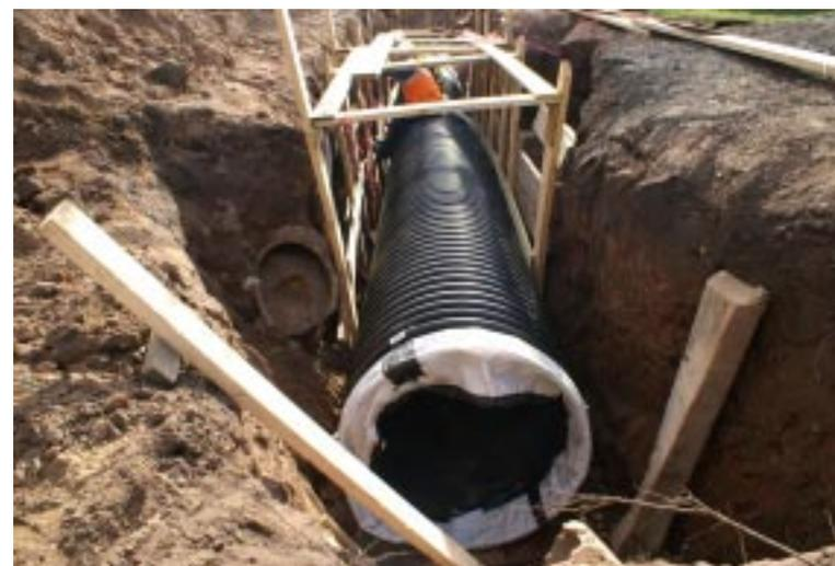
Old bywash pipe (left) and new Polypipe installed, 15-Mar-2009
