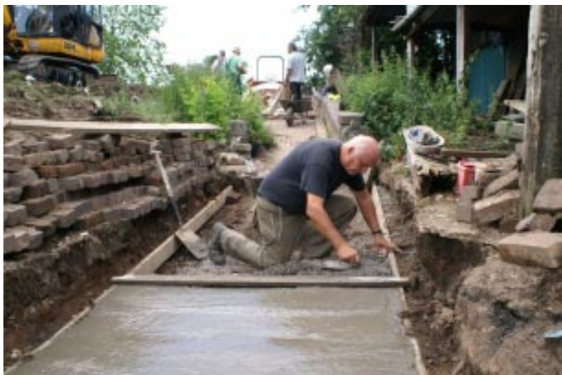
Brian Davis and crew laying new base for Lock 26 bywash.
