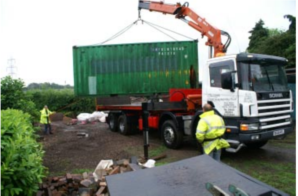
Container relocation by Chasetown Civil Engineering Ltd. (Photo by Bob Williams)
