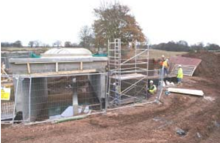
Channel showing division to support towpath at Cappers Bridge (Photo by Bob Williams)
