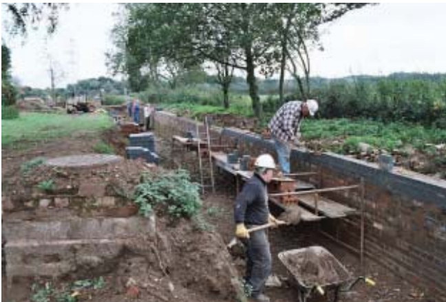
Brian adds some new courses to the rebuilt towpath wall through the garden (Photo by Phil Sharpe)
