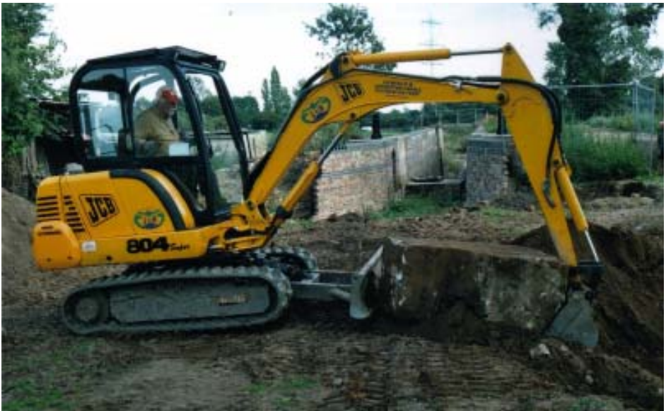
Keith using the JCB804 to drag a quoin stone from the pit above lock 26 (Photo by Phil Sharpe)
