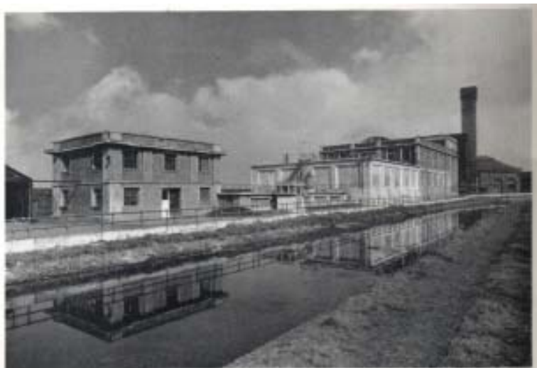
LICHFIELD FILTRATION PLANT AND PUMPING STATION
