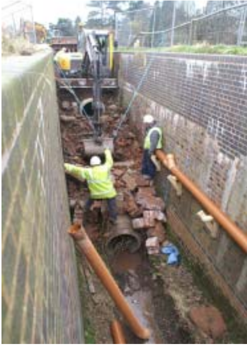
Lock 25 shaft demolition
