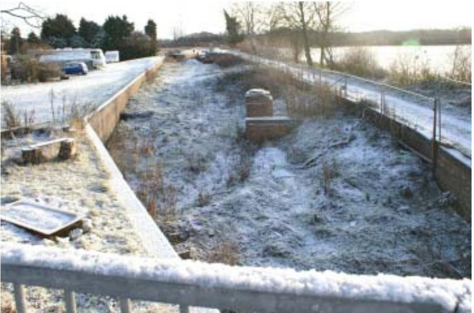
Pound 26 before the contractor moves in, December 2010
