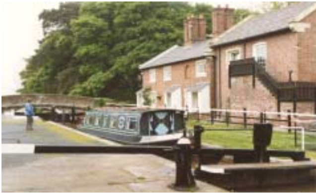
Tyrley Bridge, stairs leading up to the old clubroom, now living accommodation (photo by Penny Abbotts).
