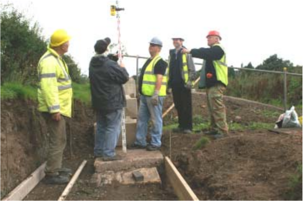
JLR start surveying the foundation level, 14-Sep-10
