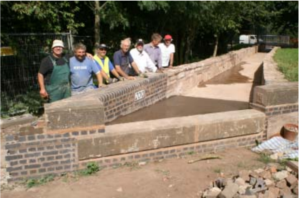
Some of the home team completing Lock 25 bywash, 21-Jul-10
