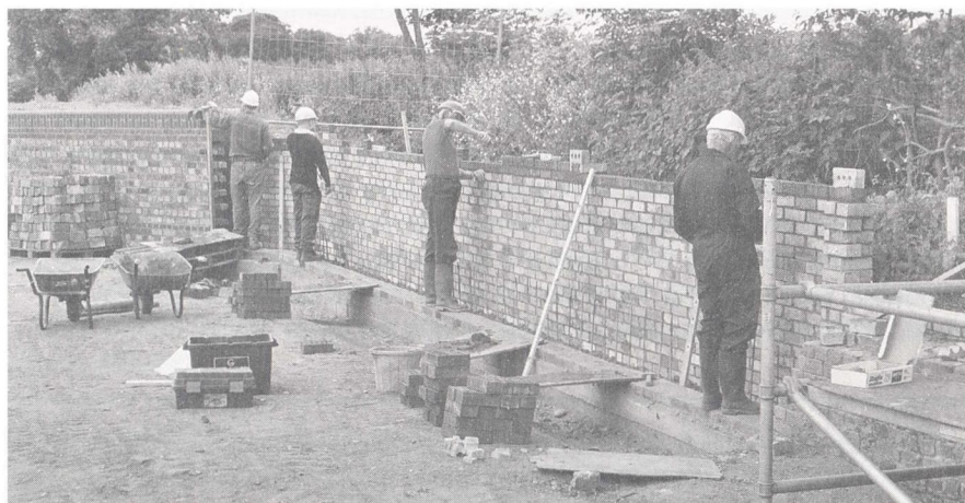
WRG BITM laying the top courses of the towpath back wall in the garden (Photo by Phil Sharpe)
