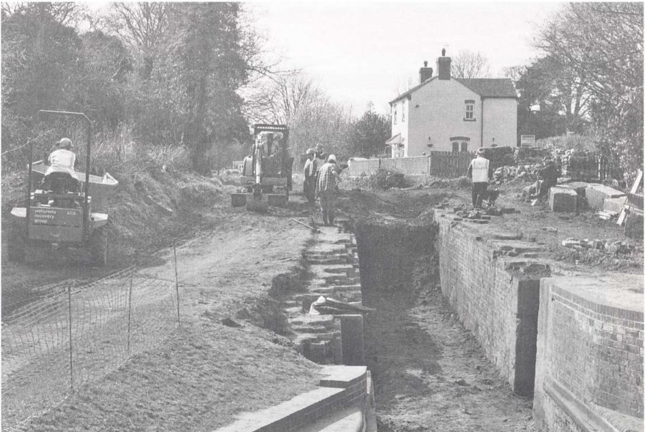
The excavated chamber of Lock 24 at the end of the Canal Camp (Photo by Phil Sharpe)
