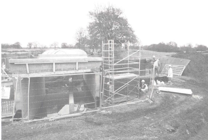
Channel showing division to support towpath at Cappers Bridge (Photo by Bob Williams)
