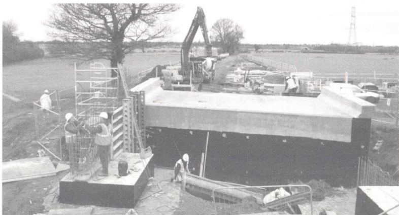
Forming foundations for wing walls at Cappers Bridge on 15 December (photo by Bob Williams)
