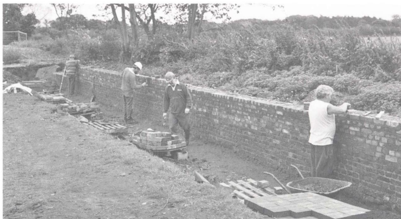
Trust and London wrg volunteers rebuilding the towpath wall (Photo by Phil Sharpe)
