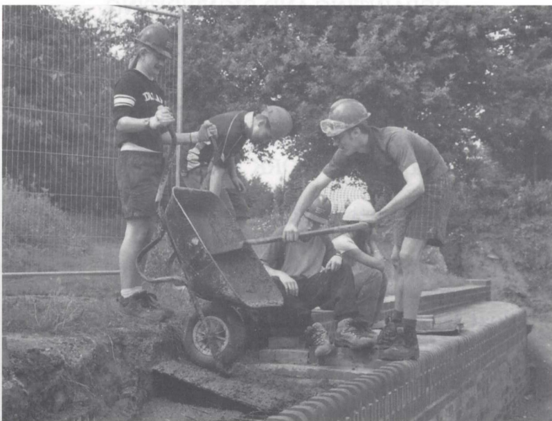
Wrg Canal Campers backfilling the wall with concrete at Lock 24 (Photo by Phil Sharpe)
