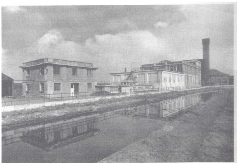
LICHFIELD RESTORATION PLANT AND PUMPING STATION
