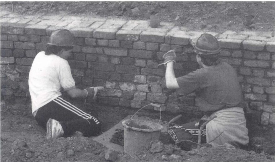
Canal Campers re-pointing the brickwork on the towpath wall (Photo by Phil Sharpe)
