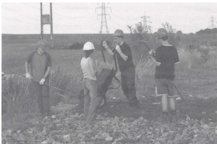
Canal campers reinstating the path at Darnford Lane with brick rubble and sand (Photo by Phil Sharpe)
