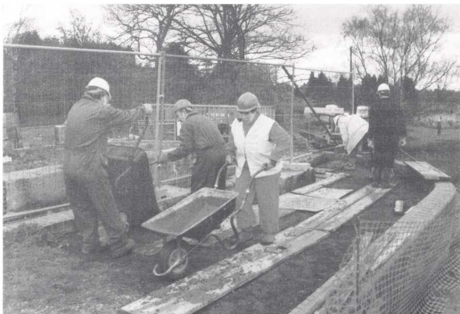
Wrg BITM barrowing readymix concrete into Lock 25 thrust block in April (Photo by Phil Sharpe)
