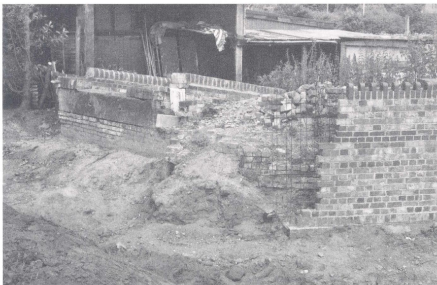
Bywash weir stone and partly rebuilt offside wing wall above Lock 26 (Photo by Phill Sharpe)
