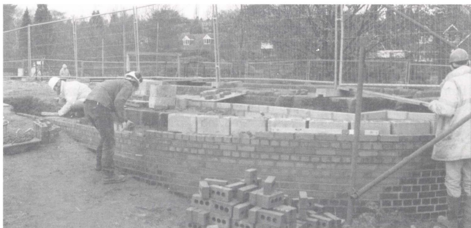
Lock 25 quadrant wall, rebuilding by LWRG/KESCRG, in December. (Photo by Phil Sharpe)
