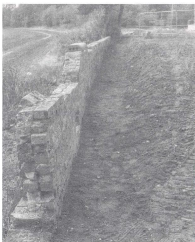
Before and after shots of Lock 25 retaining wall, Bitm laying new copings. (photo's by Phil Sharpe)
