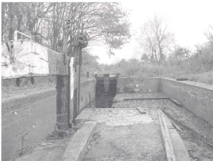
Hatherton canal Lock 2 (Photo by Bob Williams)
