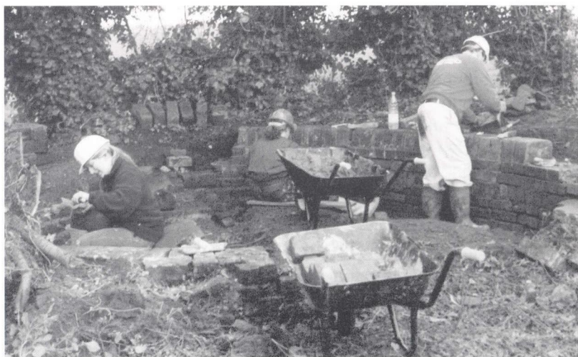
Lock 24 bywash weir consolidation by LWRG & KESCRG, in December. (Photo by Phil Sharpe)
