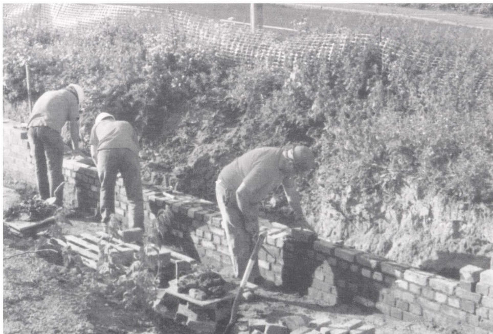
Pound 24/25 offside wall, LWRG rebuilding the gap in September. (Photo by Phil Sharpe)
