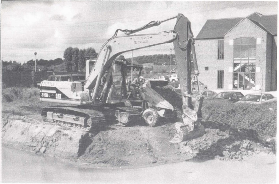
Filling the breach with clay using the dumper and CAT excavator (see page 7) (Photo by Phil Sharpe)
