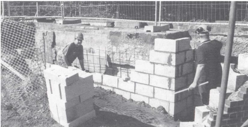
Wrg campers building the block wall for the Lock 25 thrust block in August (Photo by Phil Sharpe)
