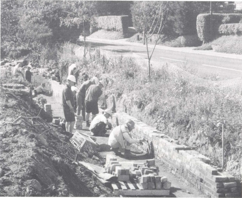
The offside pound wall takes shape during the Canal camp in August (Photo by Phil Sharpe)
