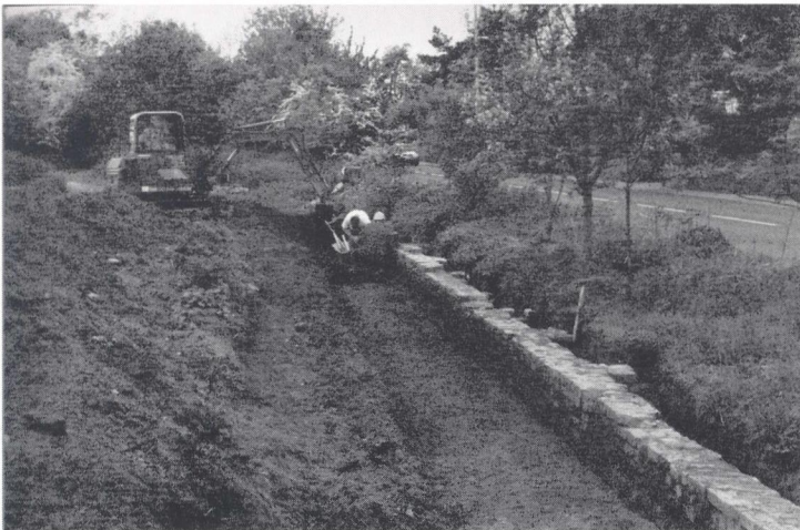
"Blue" continuing the excavation of the offside pond wall at Lock 25 (Photo by Phil Sharpe)
