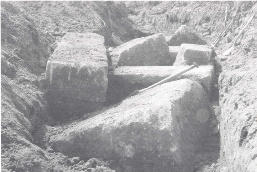
Large coping and quoin stones off Lock 24 uncovered whilst digging out the offside wall.
