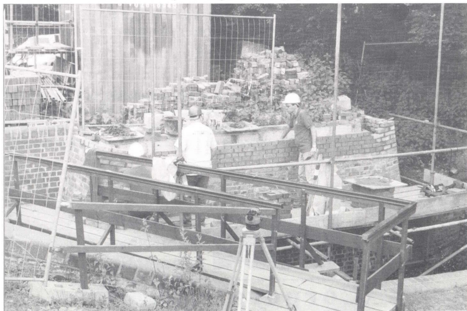
London WRG complete the bricklaying on the bridge abutment wall below Lock 25 (Photo by Phil Sharpe)
