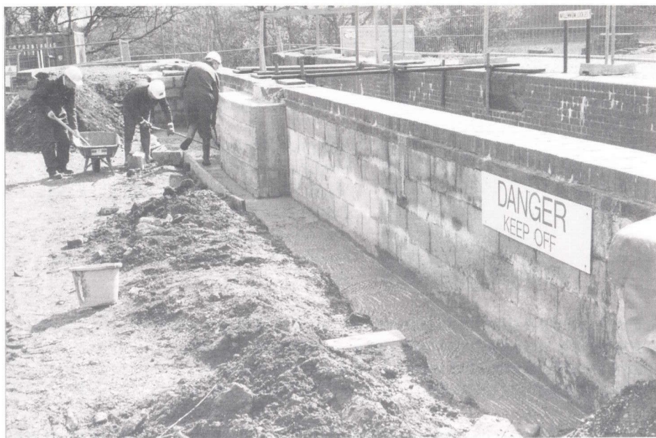
Lock 25. Northwest WRG lay concrete to seal the top of the old brickwork in April (Photo by Phil Sharpe)
