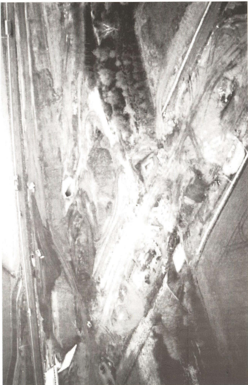
Thank you to Michael Shea, Chief Flying Instructor of the Microlight School (Lichfield) Ltd. For donating this photograph of the Lichfield Canal Aqueduct site taken on 18 th December 2002.
