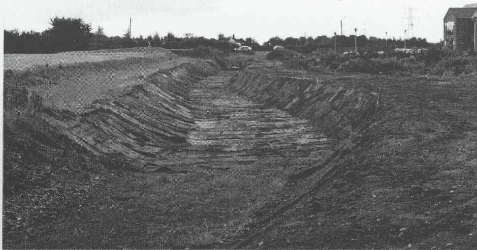
Re profiled channel at Darnford Lane, Lichfield (Photo Phil Sharpe)
