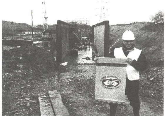
David Suchet at the site of the A5/A34 roundabout culvert for the Hatherton Canal, near Cannock.
