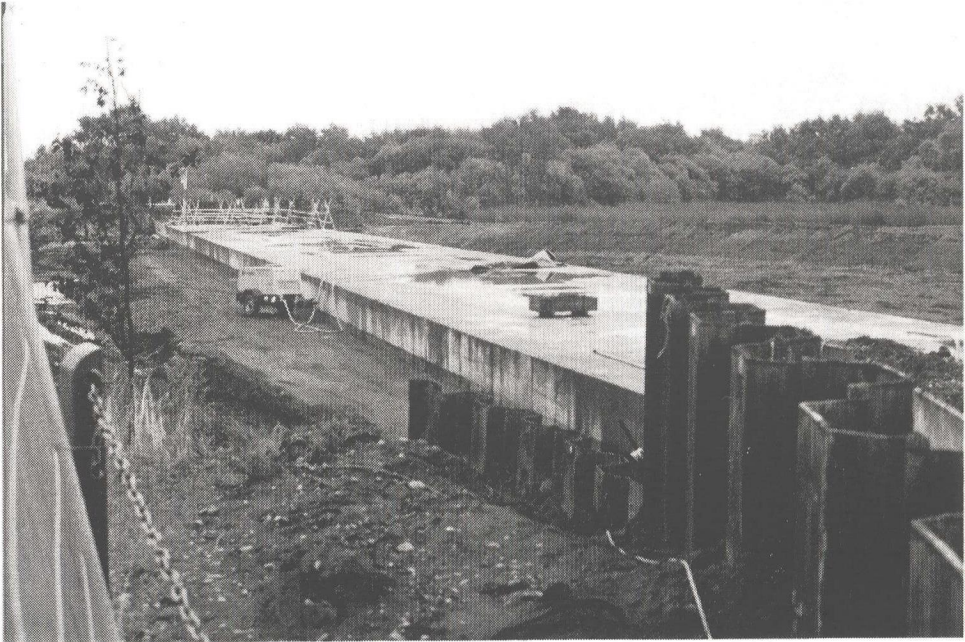
Top of completed culvert 144 under M6 Toll near Walkmill Lane, Cannock (Photo Phil Sharpe)
