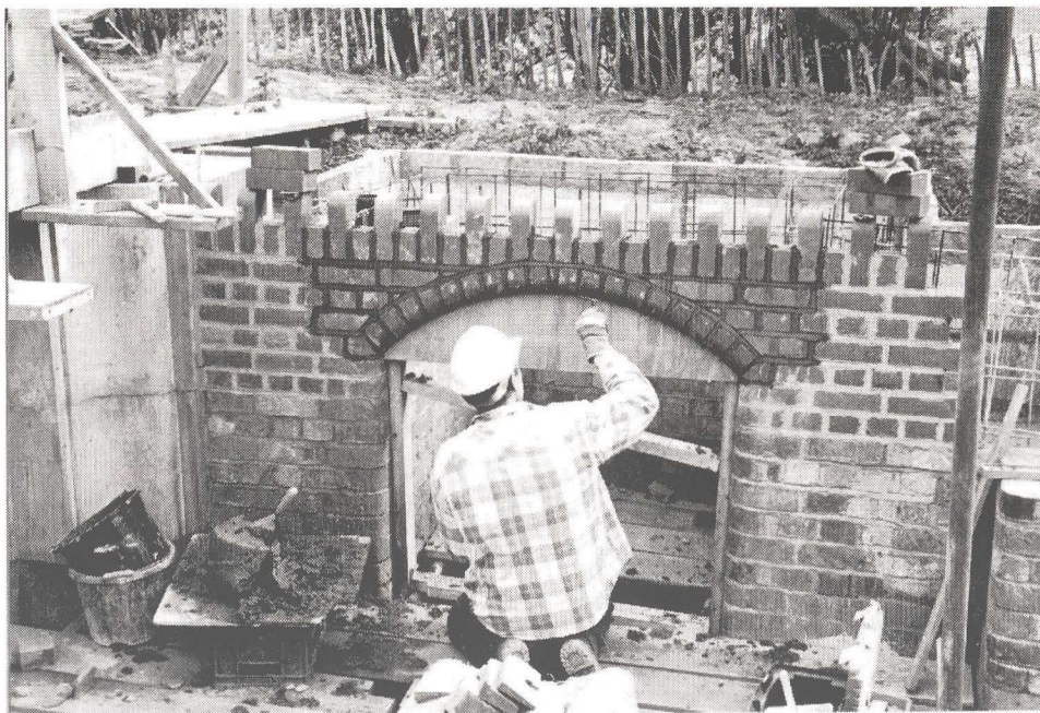
Lock 26 Tamworth Road. Peter Matthews building brick arch above the ground paddle chamber. (photo Phil Sharpe)
