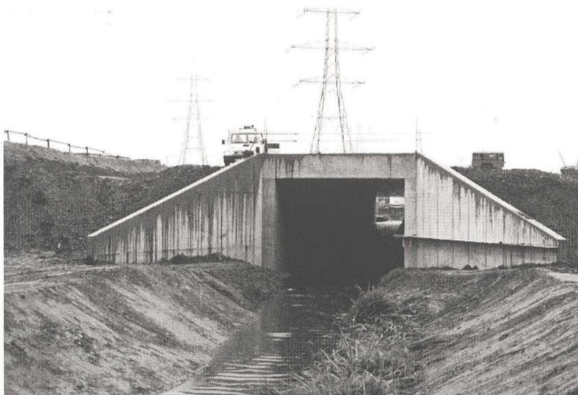
Hatherton Canal M6 Toll culvert 155 at Churchbridge complete with the Washbrook flowing through. (photo Phil Sharpe)
