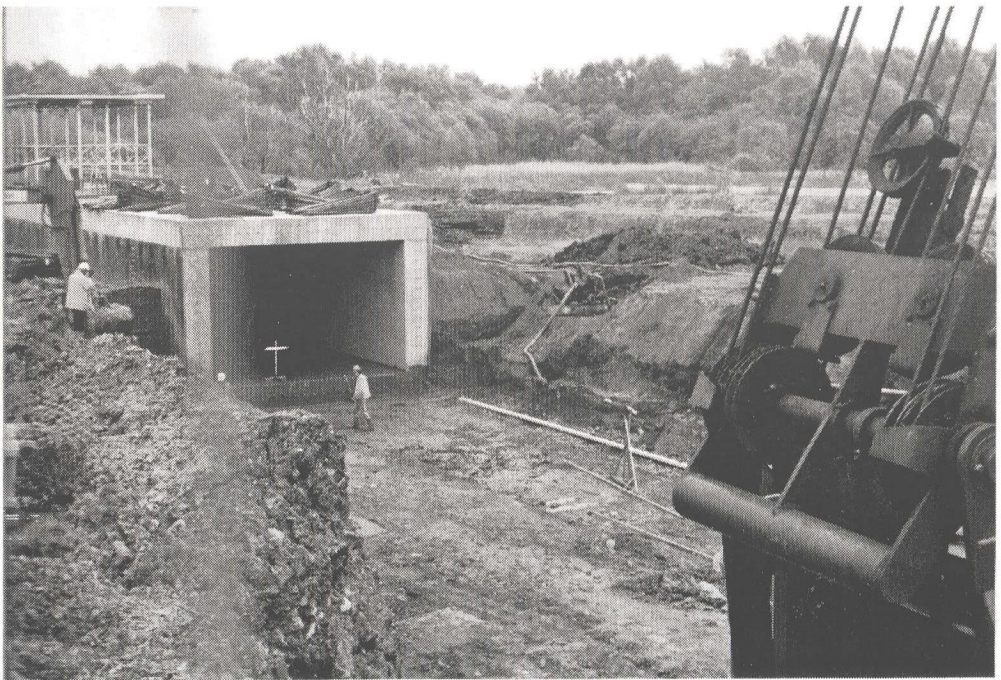
Hatherton Canal. Construction of M6 Toll culvert 144 near Walkmill Lane. (photo Phil Sharpe)
