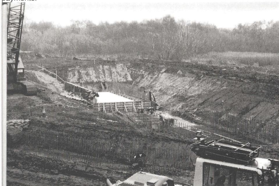
Culvert 144: The first base slab is cast and side reinforcements built 09/12/2001 (photo Phil Sharpe)
