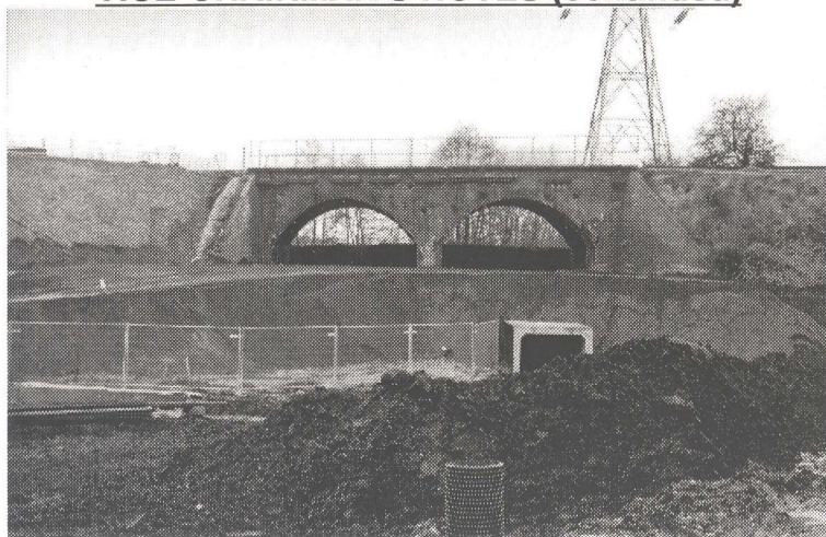
M6 Toll works burying railway bridge over Hatherton Canal at Churchbridge (photo Phil Sharpe)
