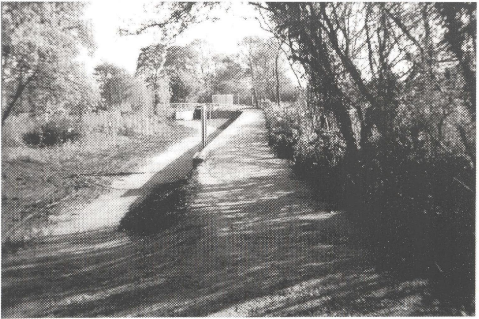
The re-instated towpath at Tamworth Road (Photo Jan Horton)
