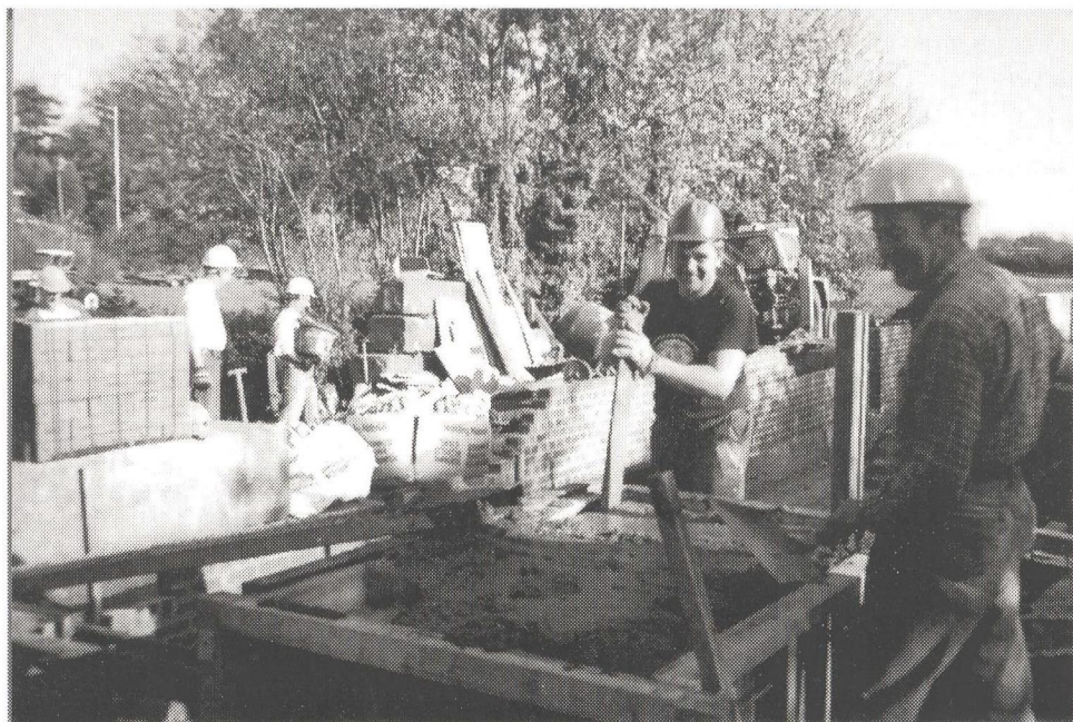
Casting new stone-work at Lock 26 in November (photo Jan Horton)
