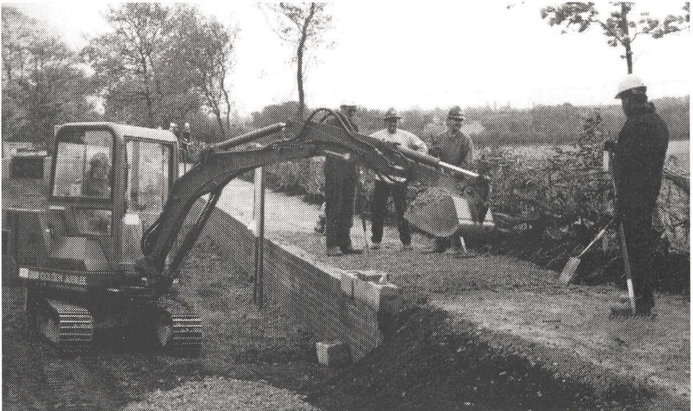
Surfacing the towpath at Tamworth Road during the WRG Canal Camp (photo by Phil Sharpe)
