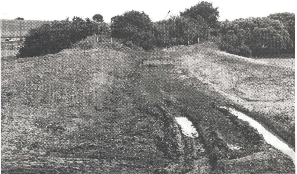
The Lichfield Canal embankment at Crane Brook, cleared of vegetation where the BNRR will cut through and the new aqueduct is required. (photo Phil Sharpe)
