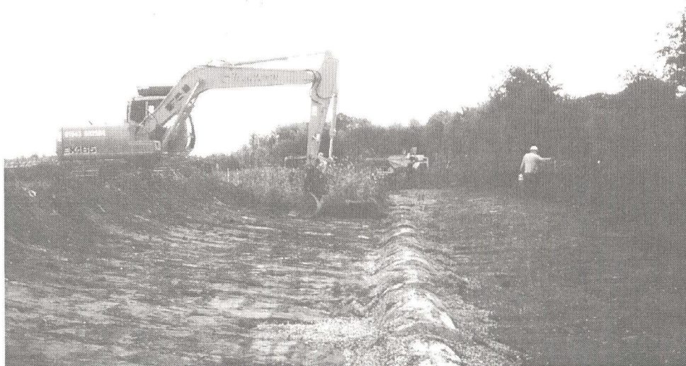
Chasetown Civil Engineering's donation of 16-ton excavator and driver for a week-end, being used to clear the channel from Lock 26 towards the A38 (photo Jan Horton)
