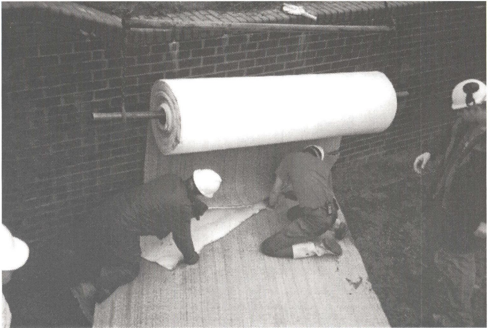
More bentonite lining being laid at Darnford Lane (photo Jan Horton)
