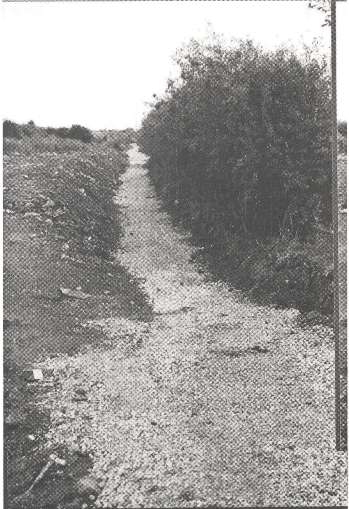
Fosseway towpath surfaced
