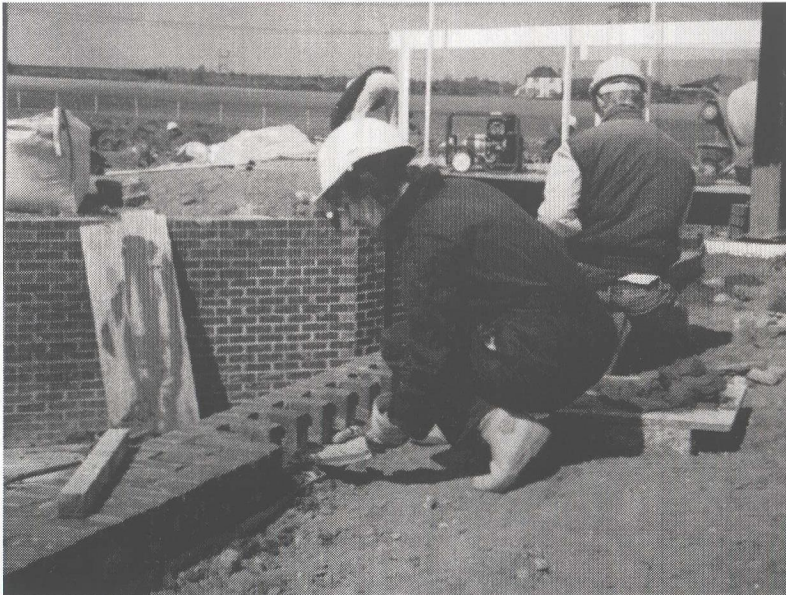
Newbury Working Party Group Laying coping bricks at Darnford Lane
