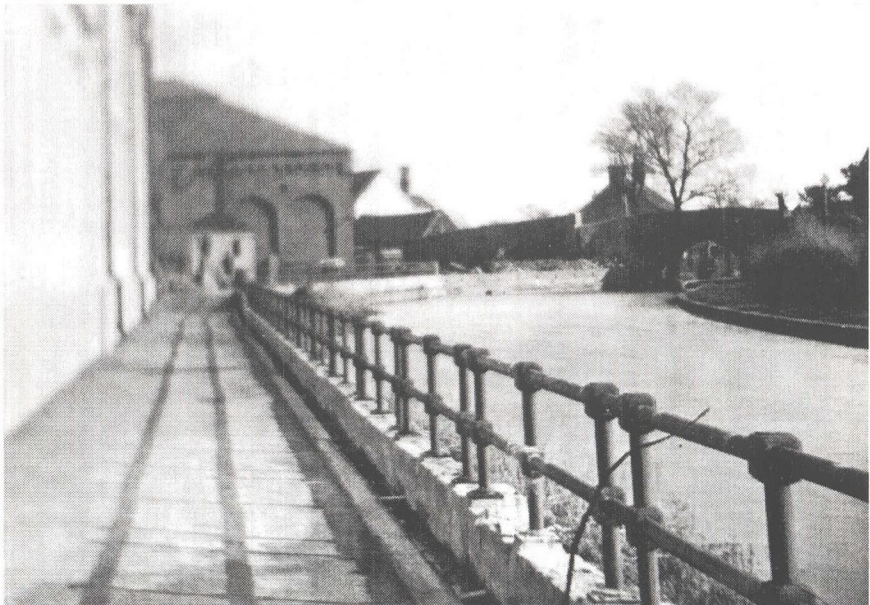
The canal alongside the now demolished filtration plant and boiler house
